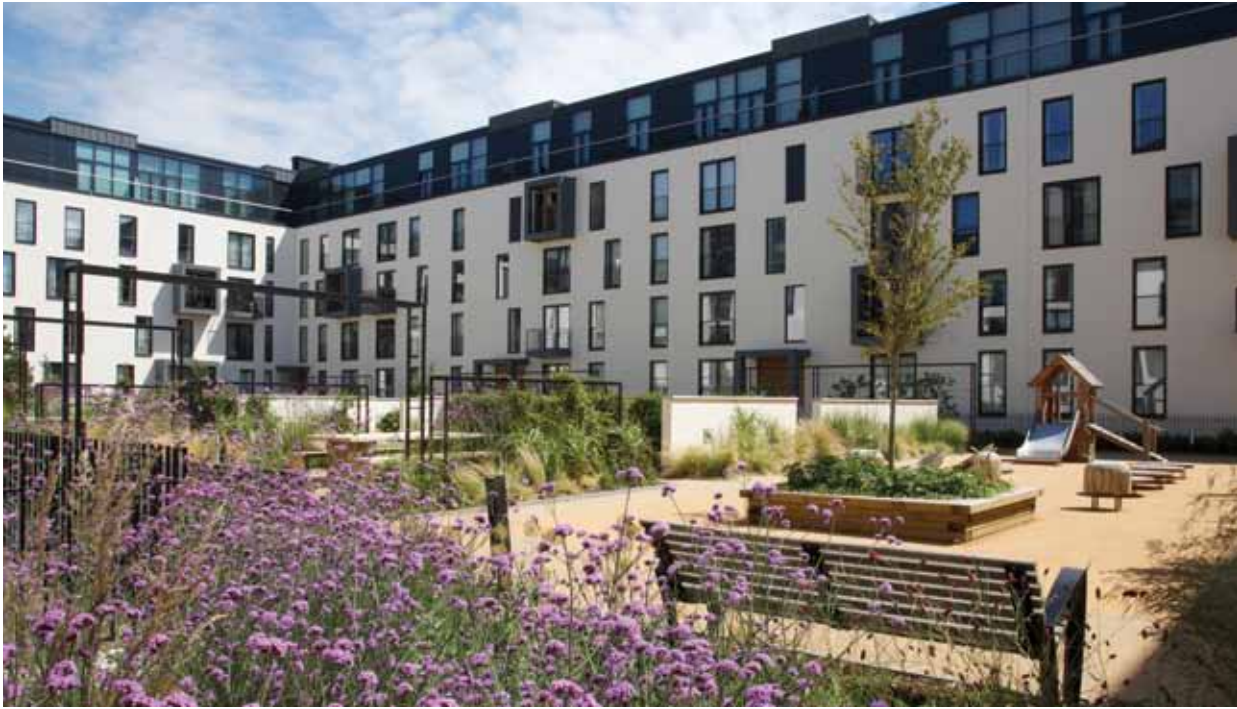
Phase 1 Courtyard Gardens – completed
